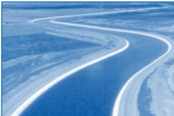
California Aqueduct delivering water to Southern California
