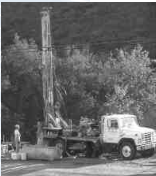
Geotechnical drilling along tunnel route.
