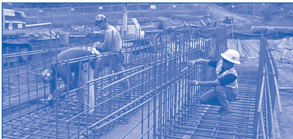
**Carlos (right) inspects reinforcing steel for a concrete pipe encasement**
