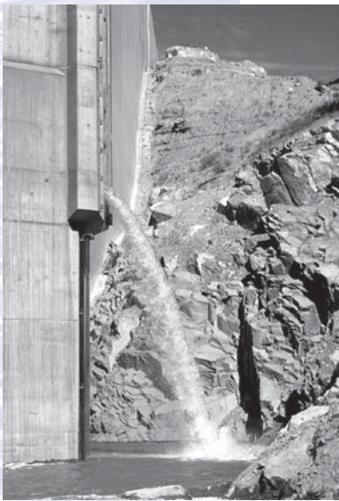
The Olivenhain Reservoir is filled with imported water.
