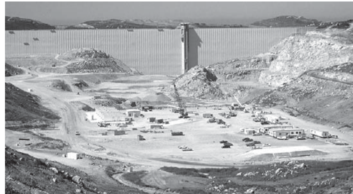
Water Authority completes construction on the Olivenhain Dam.
