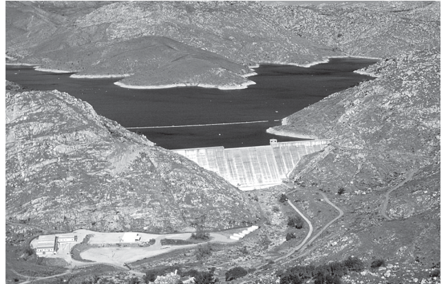
The San Vicente Dam currently stands at 220 feet.
