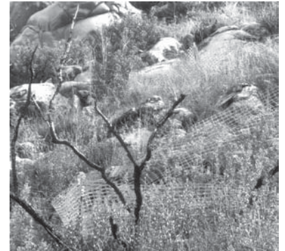
Fencing protects sensitive plant species from potential impacts at a construction site.
