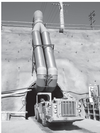
The Lake Hodges tunnel is now more than 2,000 feet long.
