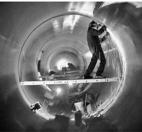
Each of the 148 pieces of pipe were welded together to form the pipeline.
