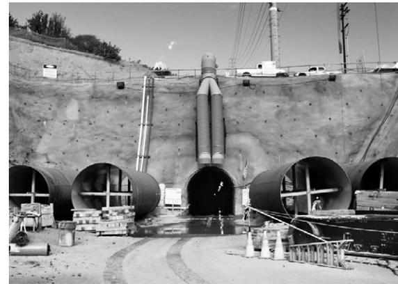
*Pipe sections 10 feet in diameter are inserted one by one in the tunnel and welded together.*
