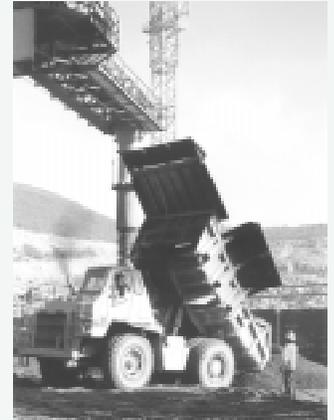
**7.** A spreader follows closely behind each dump truck and moves roller-compacted concrete evenly over the dam.
