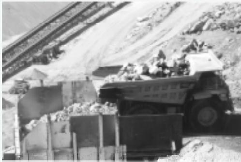
**6.** Each dump truck drives to the section of the dam being worked on and dumps its load of roller-compacted concrete.
