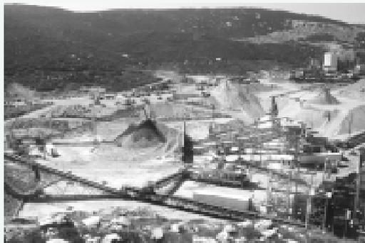
**3.** Once crushed, rocks are stored in stock piles until they are conveyed to the batch plant.
