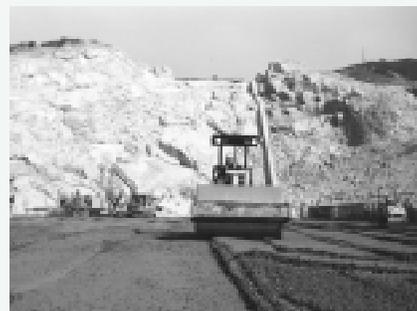
**8.** Large 10- and 12-ton vibratory rollers follow the spreaders and drive on top of the roller-compacted concrete to compact it to a 12-inch layer, known as a lift.
