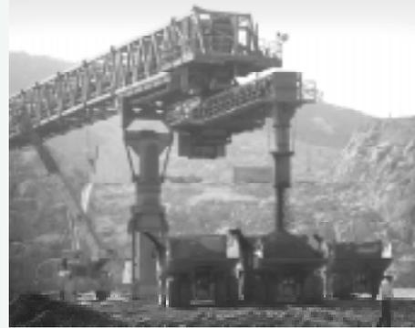
**5.** Roller-compacted concrete from the batch plant is loaded into dump trucks on the dam's surface.
