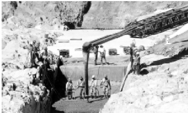
*Olivenhain Dam construction workers fill large holes in the foundation.*
