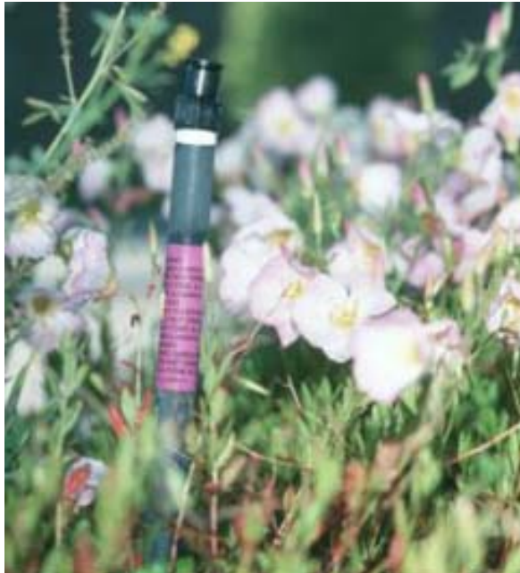
Purple fixtures are installed throughout the county where recycled water is used for irrigation.
