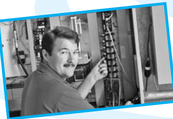
Computers assist employees in monitoring the District's Water System
