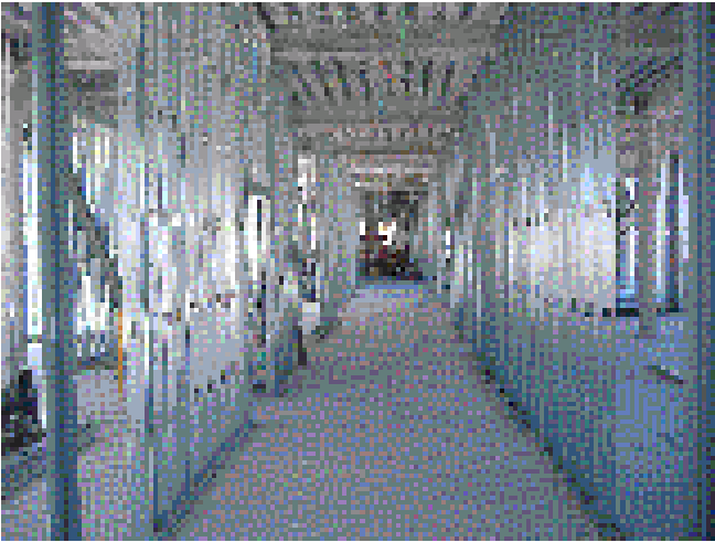
This is an Interior hallway with framing in one of the patient "neighborhoods".
