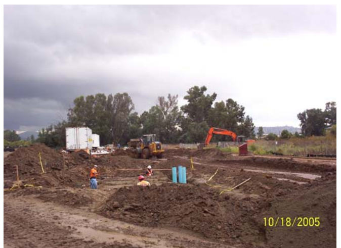
Storm Drain Work Close Up
