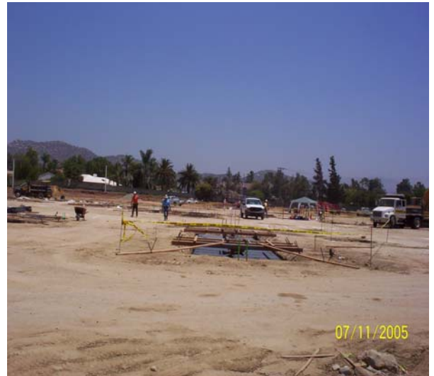
Northeast Site View
