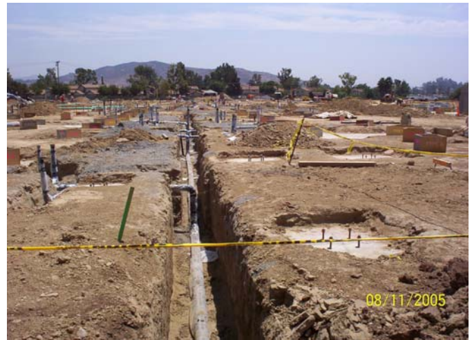
Underground Plumbing Lines
