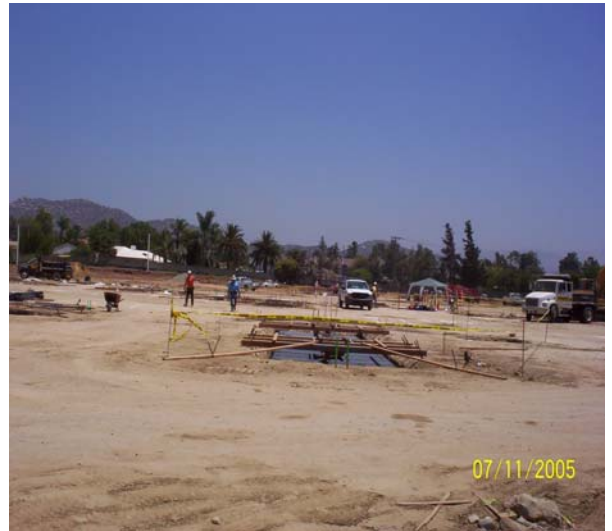
Northeast Site View
