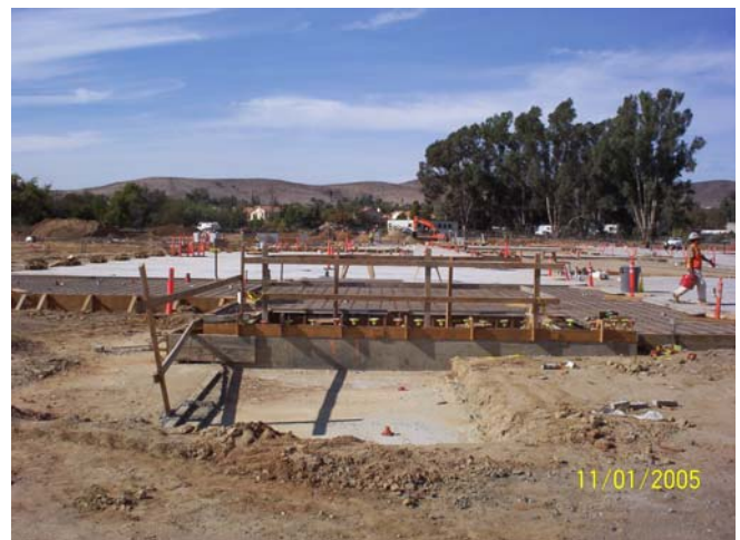
Partially Completed Slab
