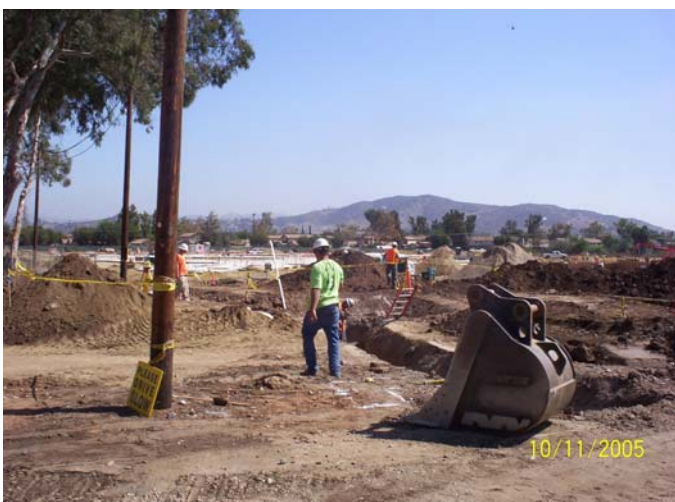
Northwest Corner View
