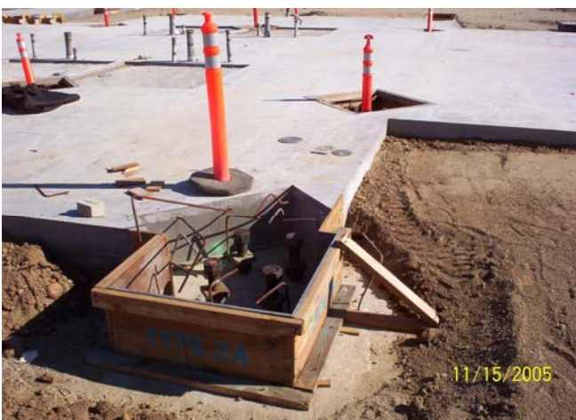
Building Corner Post
