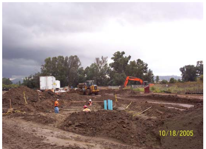
Storm Drain Work Close Up
