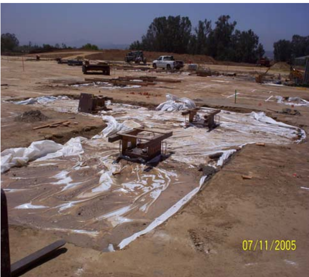
View of the support Footings
