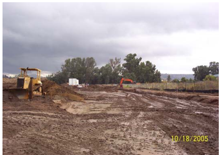
Park Center Drive Storm Drain Work
