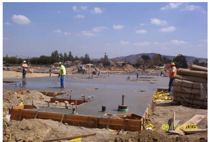
The Concrete Is In!
