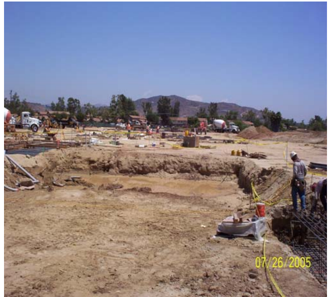
Loading Dock Grading
