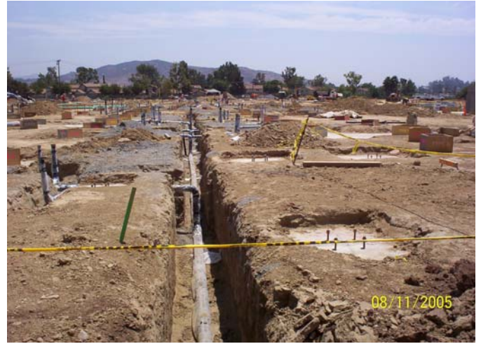
Underground Plumbing Lines
