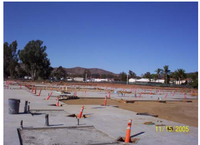
View of Foundation
