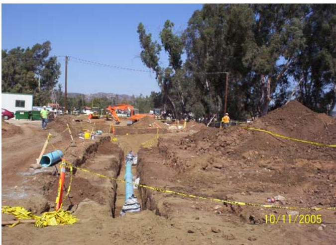
Water Lines Under Park Center Drive
