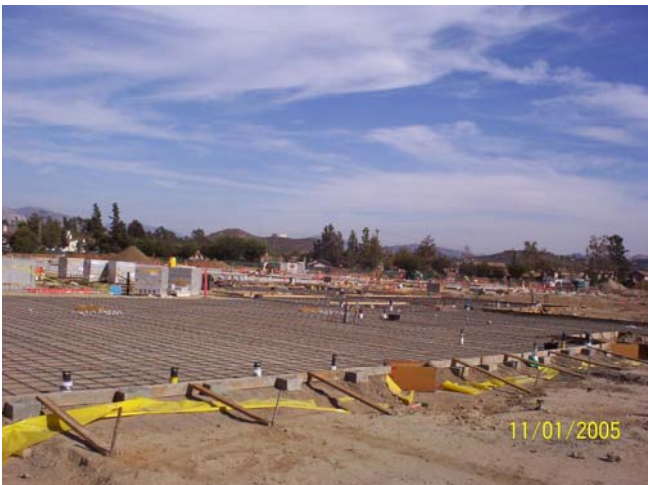
Foundation Prep For Concrete
