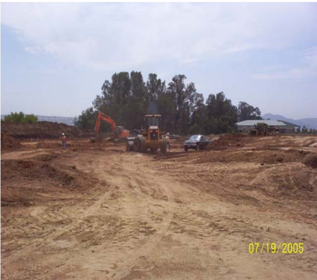
Parking Lot Grading
