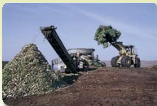
Yard waste is ground into mulch and compost at the Miramar Landfill.
