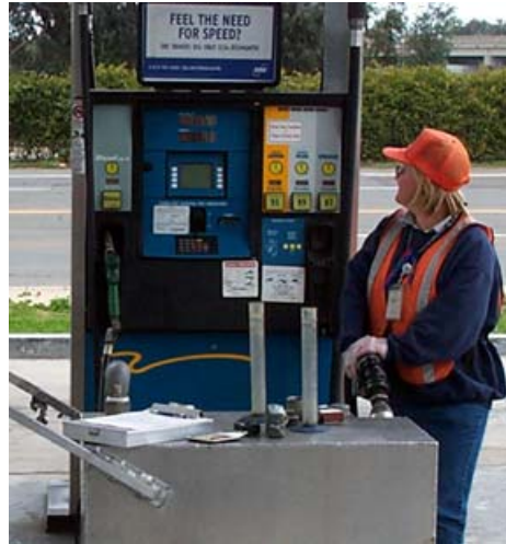
Compliance inspectors ensure that vapor recovery systems are working properly.
