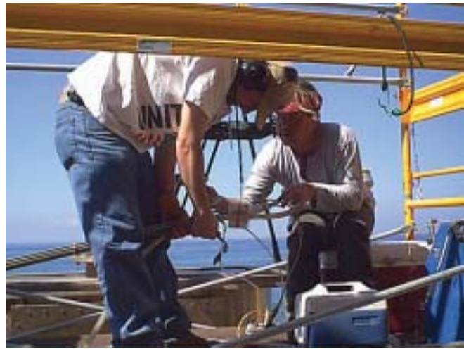
District chemists set up test equipment for a particulate test of a diesel engine at the Pt. Loma Wastewater Plant.
